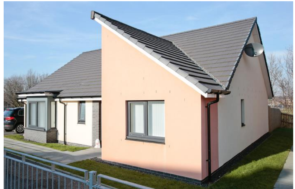
Wheelchair Bungalow, Link Housing Development, Tannahill Crescent, Johnstone
