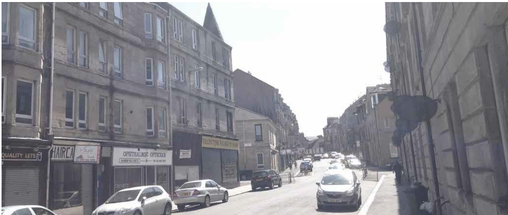
Well Street view south - Existing
