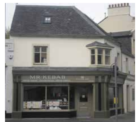
Figure 50: 36 Causeyside Street (restored)
