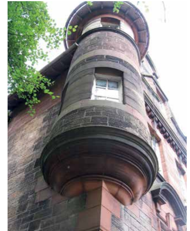
Former Territorial Army Building
