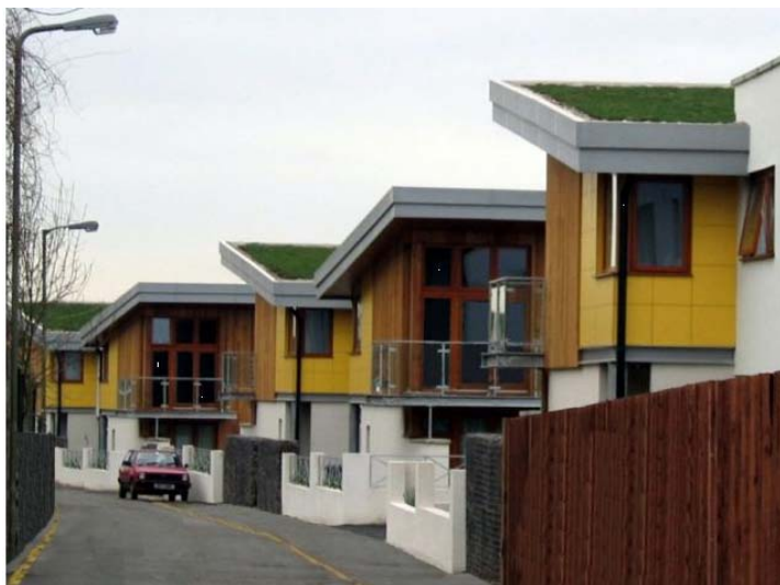
Photo 1 – Green Roofs on a Modern Development
