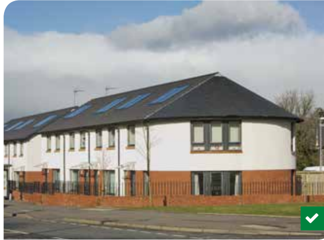
The council development at Barrhead Road, Paisley uses solar thermal panels to help with heating water and reduce energy bills for residents.
