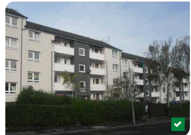
These flats at Maple Drive, Johnstone have been refurbished in order to provide a higher level of energy efficiency. The external wall insulation can reduce energy consumption by up 25%.
