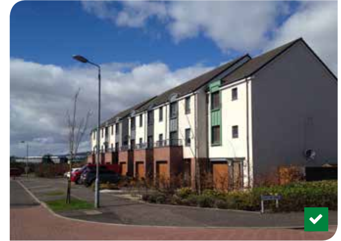
Terraced and flatted properties tend to have higher energy performance than detached properties. These townhouses in Crofton Avenue, Renfrew have a higher level of energy performance because less external walls being exposed to the elements.
