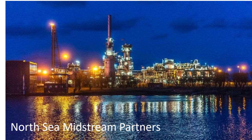
The St Fergus Gas Terminal is at the centre of the Acorn Project
