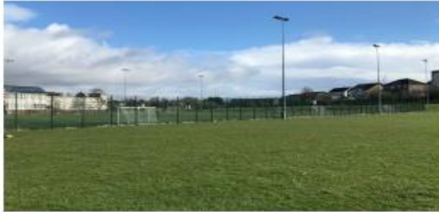
EXISTING ABACUS 15m HIGH LIGHTING COLUMNS
