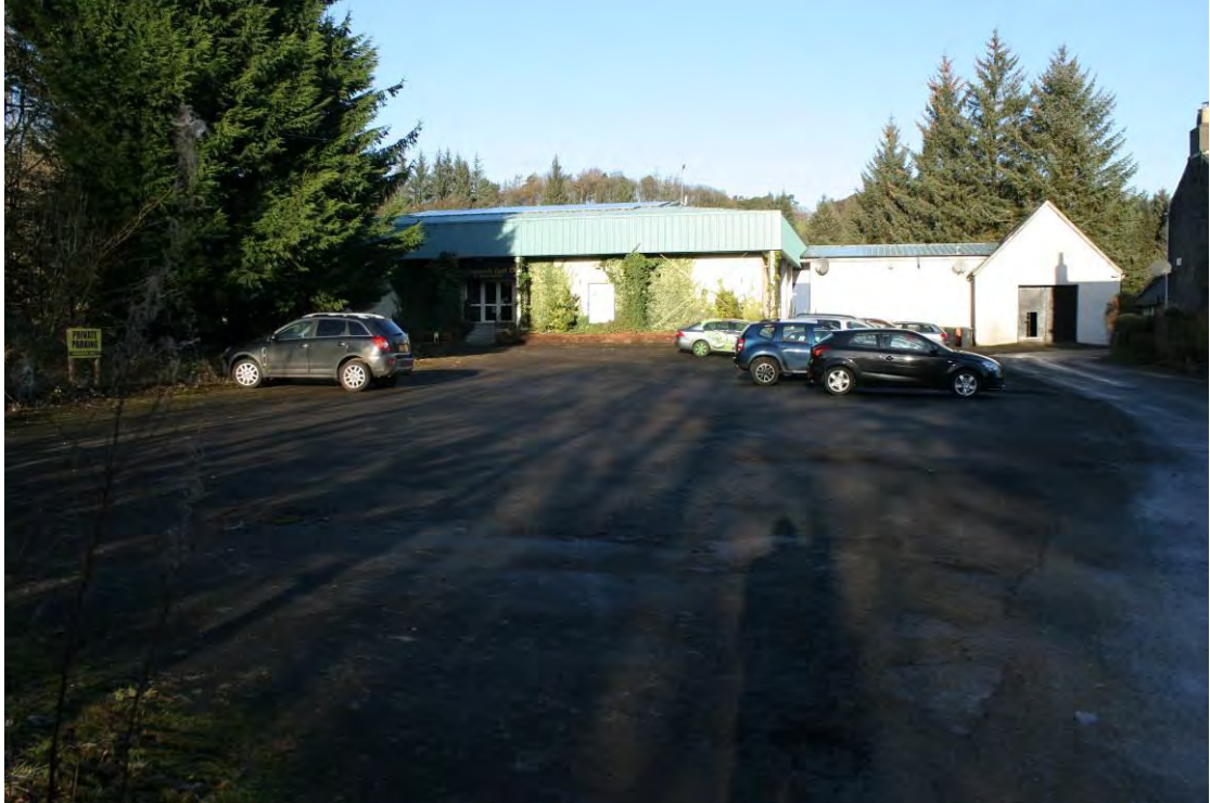
Golf club house building seen from the south.
