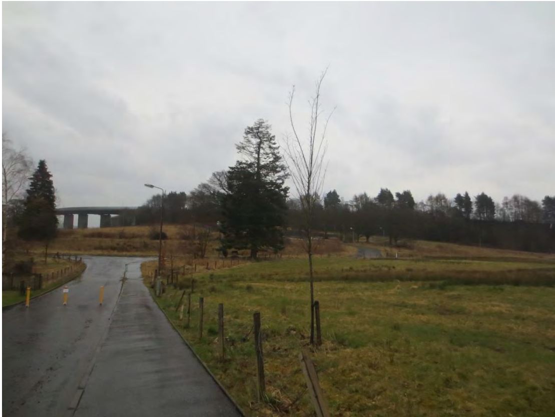
View south from Nursery Avenue to the Erskine Bridge.
