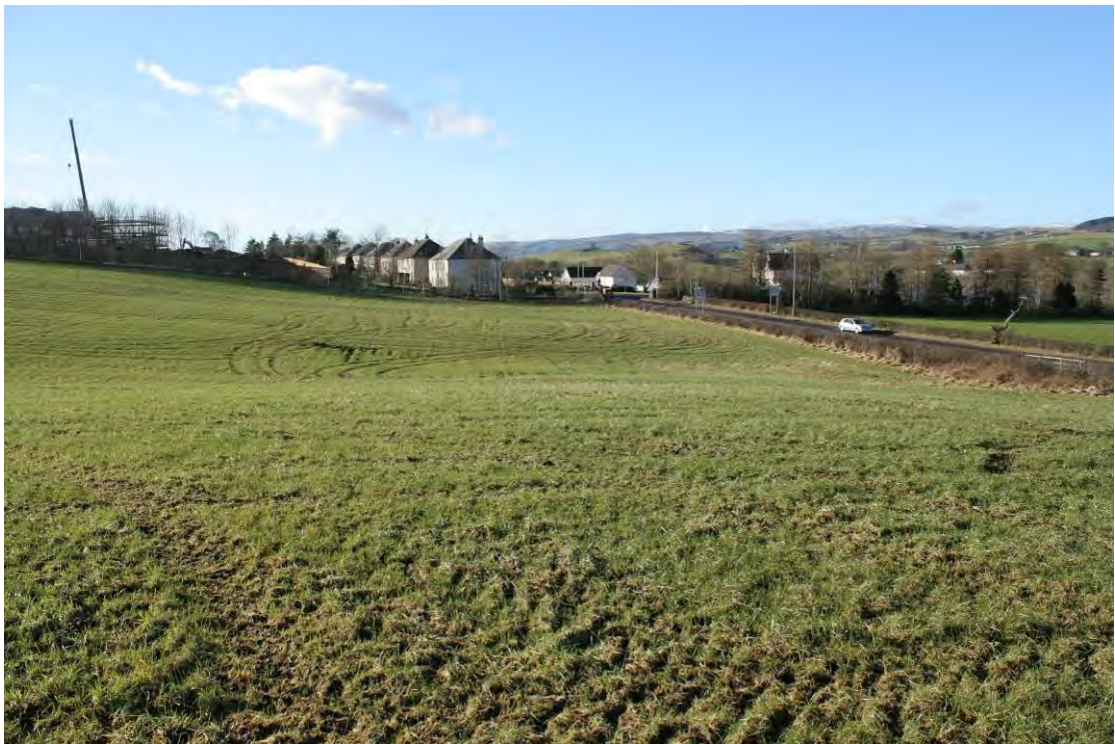
View west from the site to the settlement edge, including new housing under construction.
