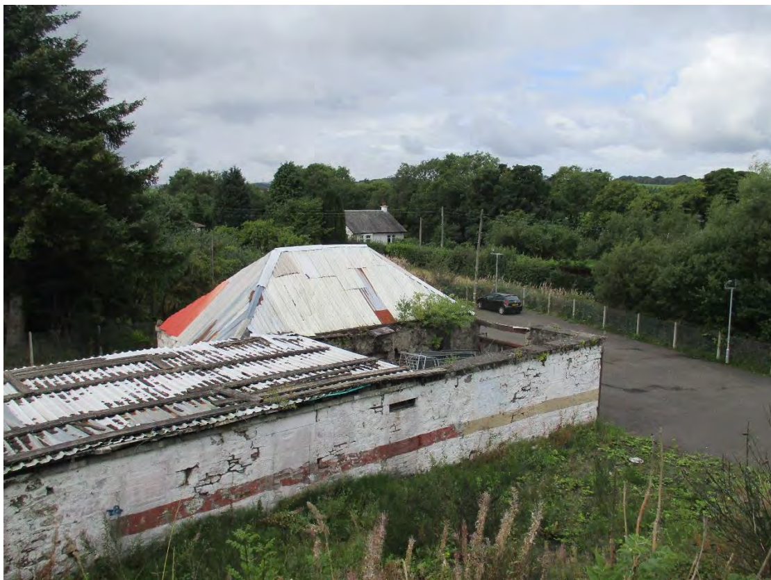
Derelict buildings and houses at the eastern part of the site.
