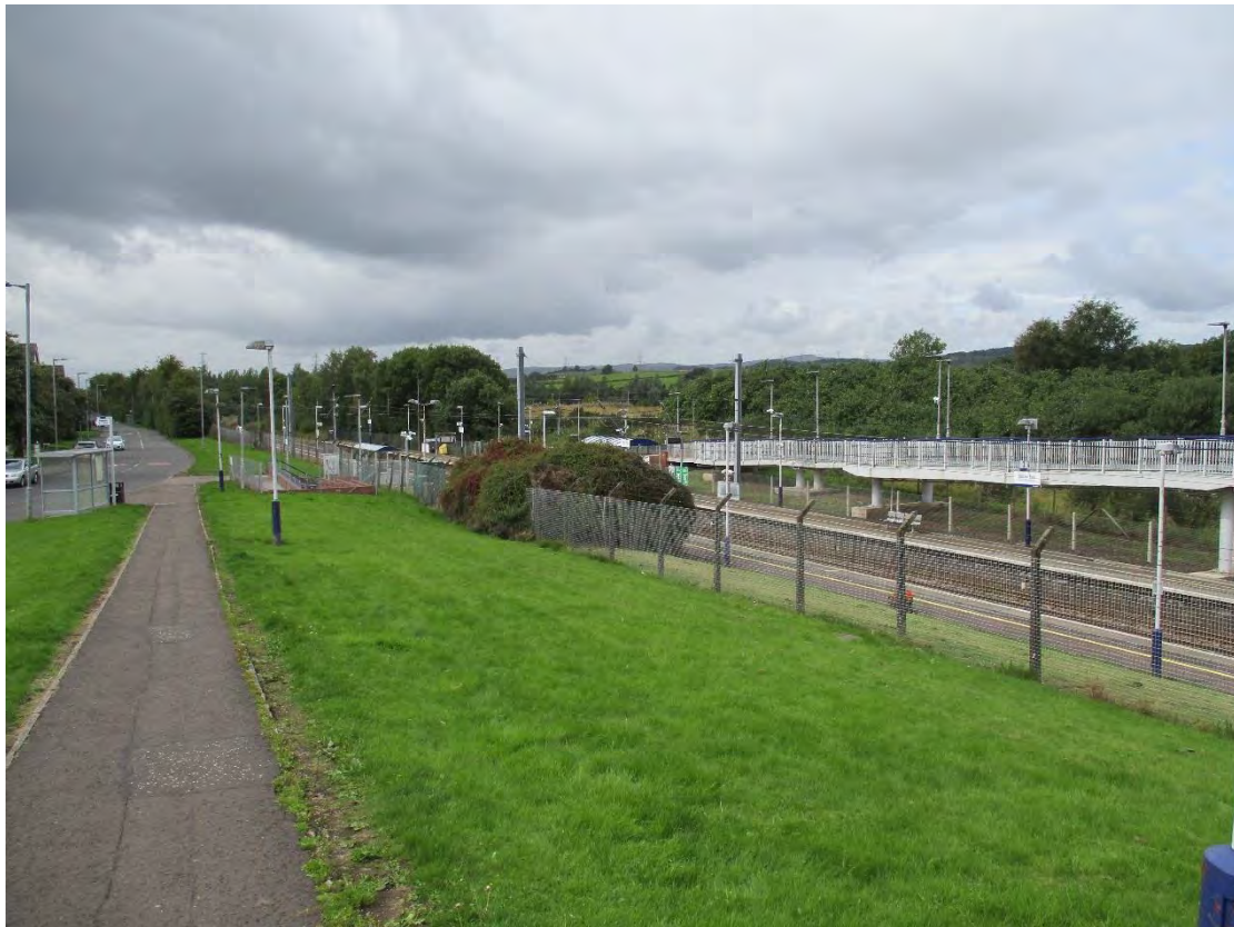
Milliken Park station and the railway line along the southern site boundary.
