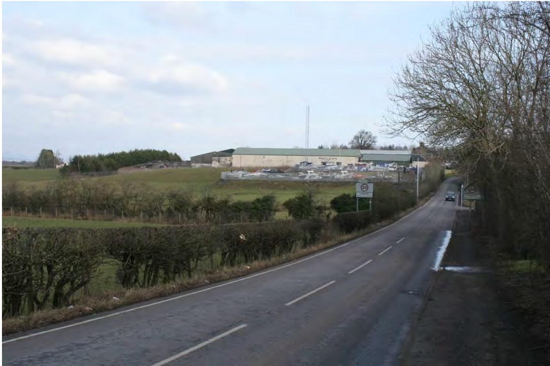
The site as seen from Darluith Road on the to Linwood from the west.
