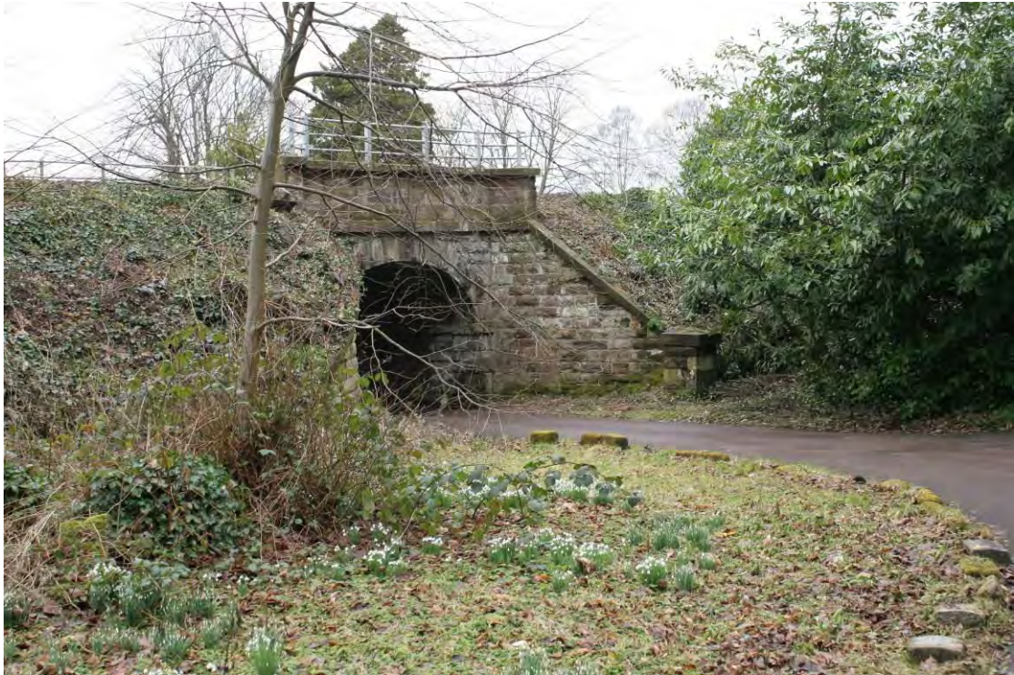
Access to the site beneath the railway line.
