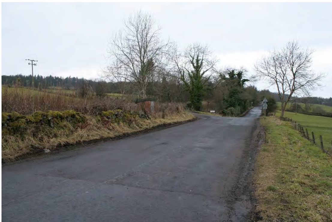
Old Greenock Road looking west along the southern site boundary
