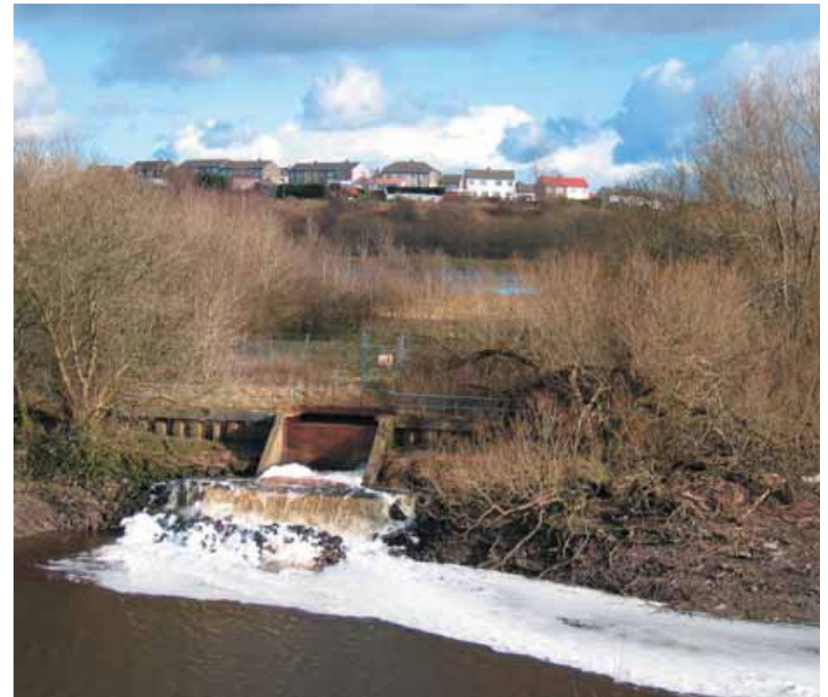
Effluent discharge to White Cart from Abercorn sewage treatment works
