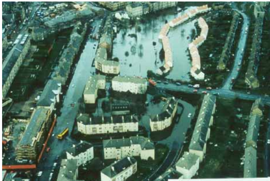
Sewer flooding from blocked drainage culvert Stockholm Crescent (1994)
