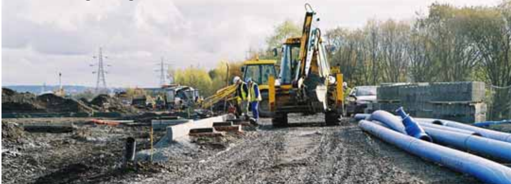
Road drainage, Kings Inch Road, Renfrew
